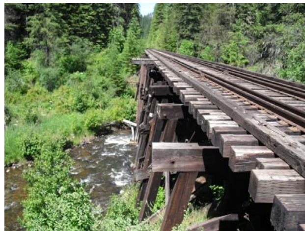
Orofino Creek Rail Bridge. Photo: Monica Walker
