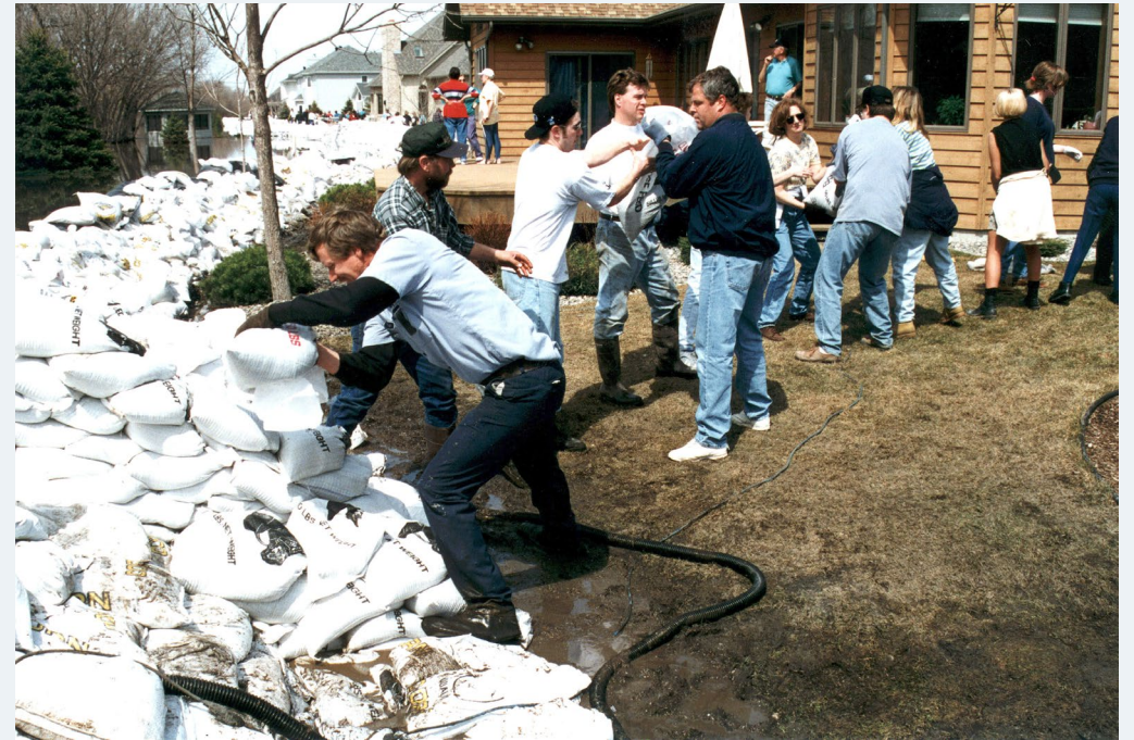
Residents of Fargo, ND, build up a sandbag levee to fight the rising waters of the Red River. Image by David Saville/FEMA via National Archives.
