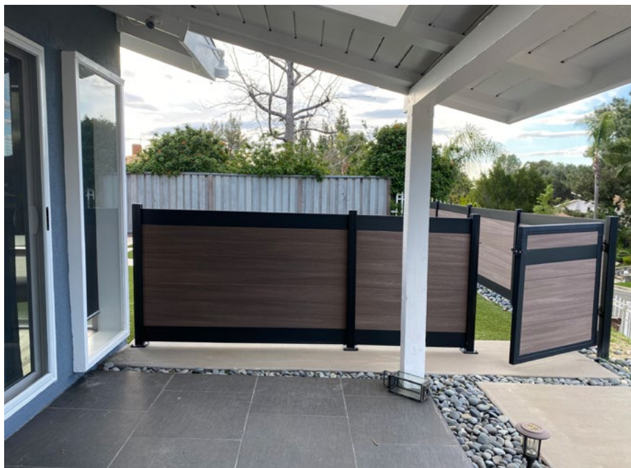
Figure 8: Noncombustible fencing should extend 5 to 10 feet from the home (Photo: Shearman Builders)
