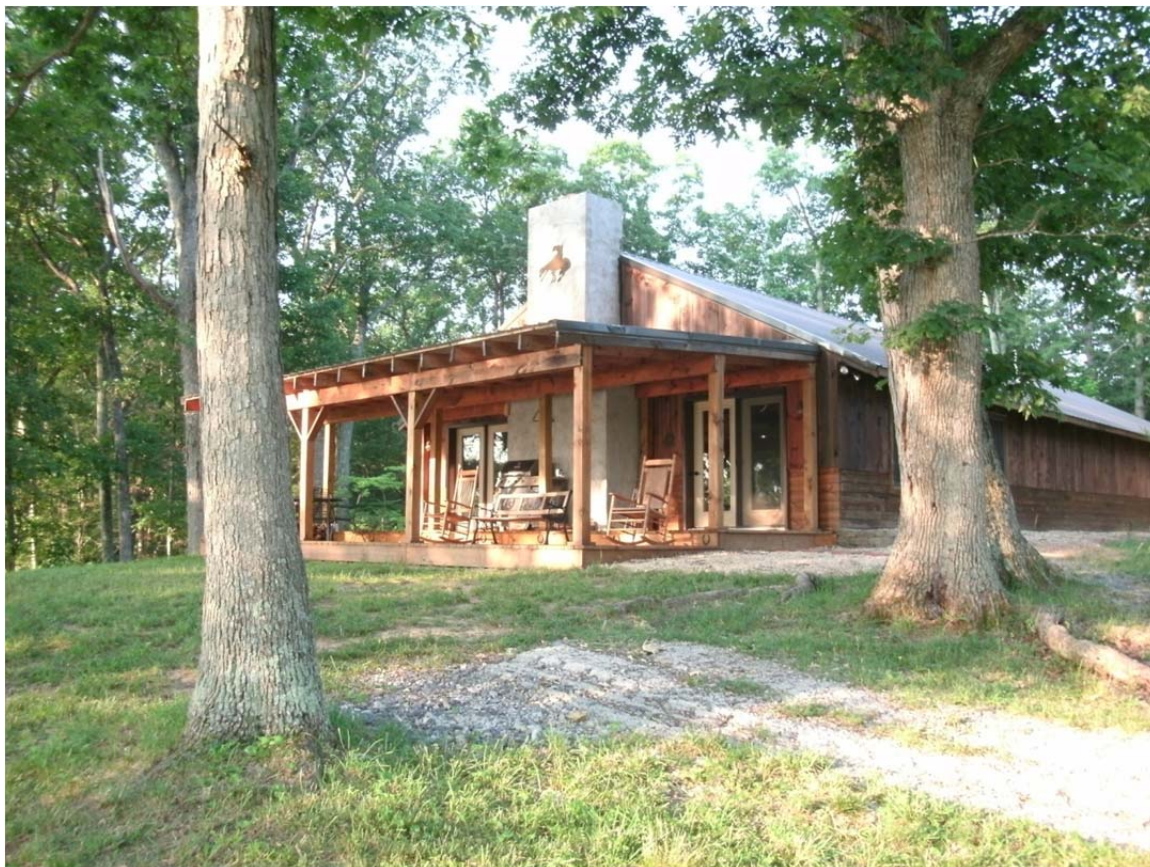
Figure 6.4: Photos of North Mountain Outfitters Bunkhouse
